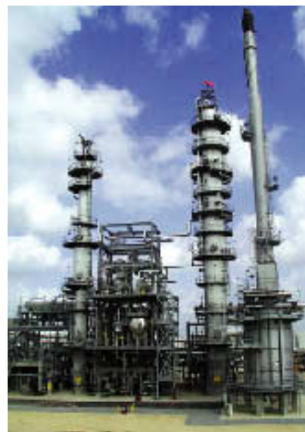
Motiva's plant in Port Arthur, Texas uses the CDHDS process to produce low sulfur gasoline.
